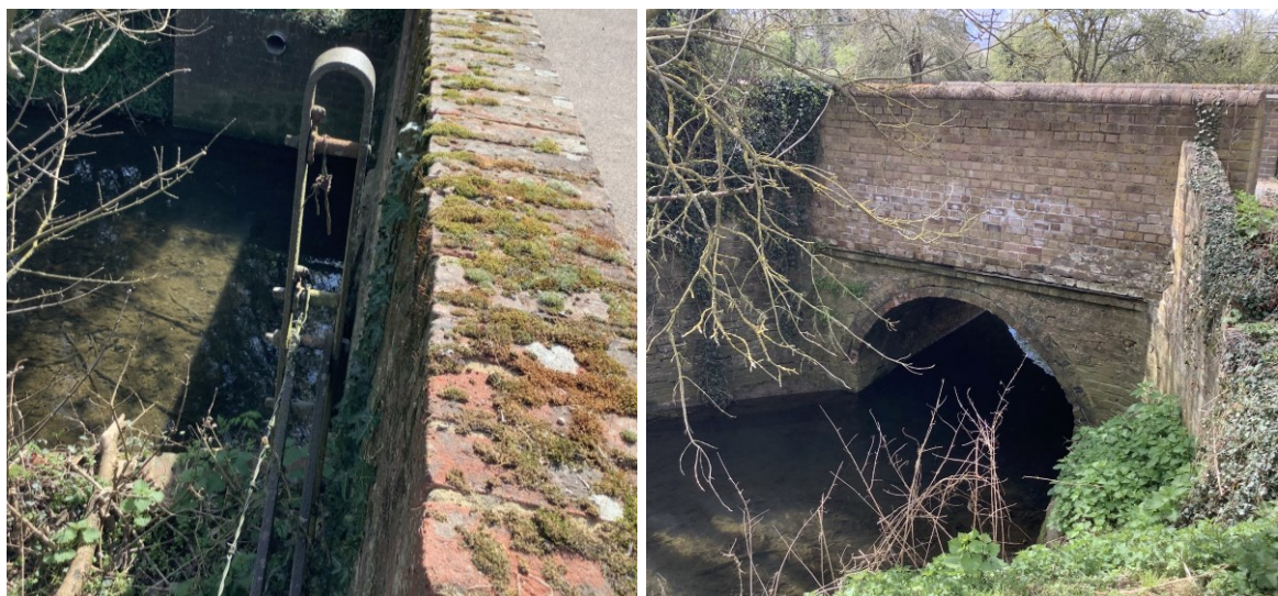
Figure 29: Weir (left) and Bridge (right), High Street
